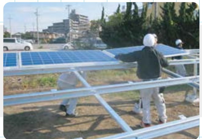
08 太陽能板安裝 Fixing Solar Panels
