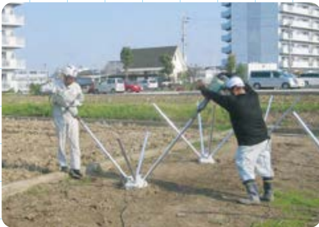
04 釘入鋼管 Driving Steel Pipes
