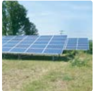
距離地面較近的施工案例 Height near to the ground level
