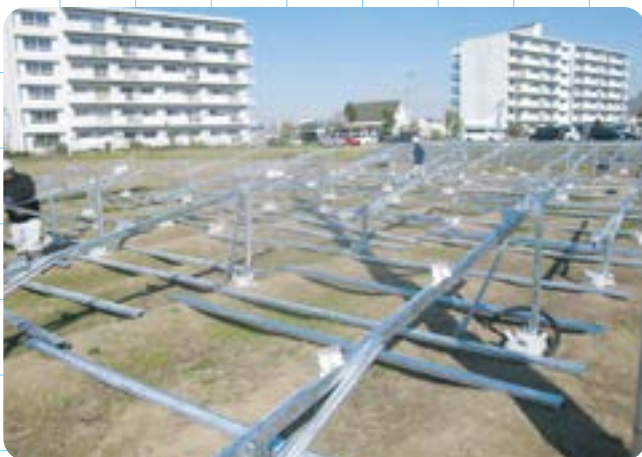
07 支架組裝 Assembling Mountings
